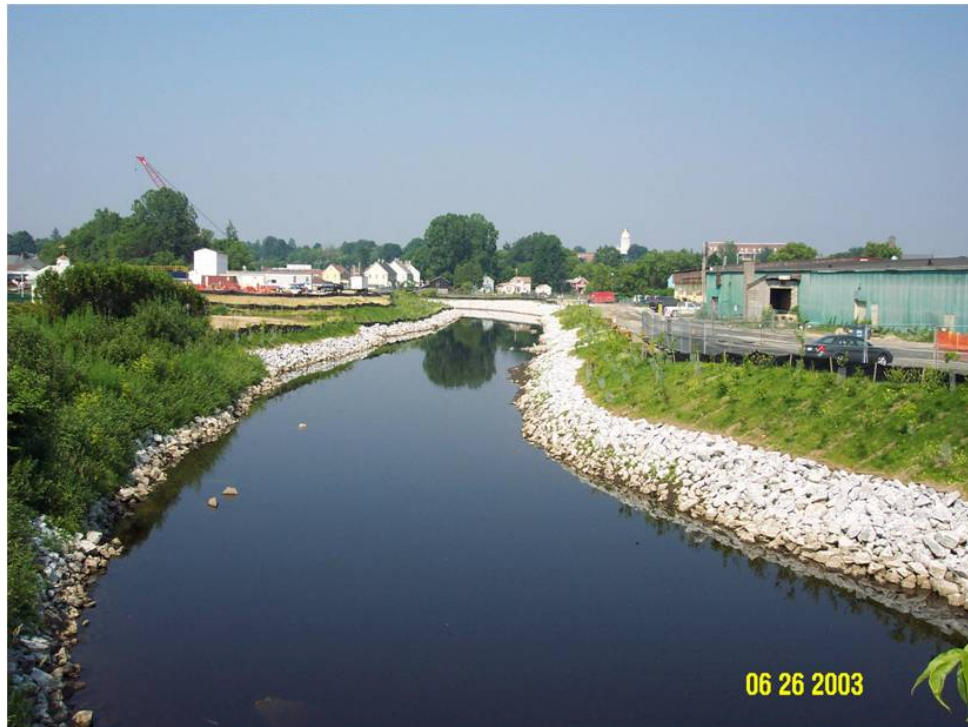
1 1/2-Mile Reach: Lyman Street, Looking Downstream. Immediately After Remediation
